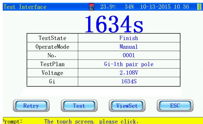
Fig. 3.3.1-2 More than 2 poles voltage and battery conductance test
